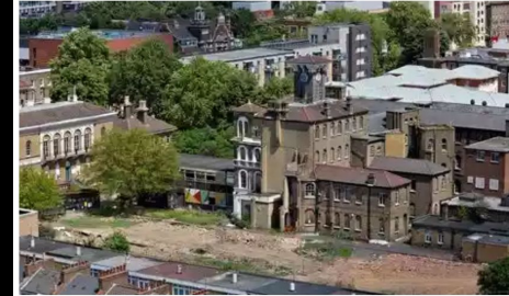
The former St Clement's hospital in Mile End, east London, where London's first community land trust is being built.
